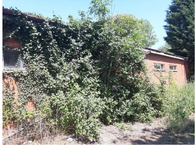
Plate 9.14: Southern Elevation of the Building with Dense Ivy Coverage
