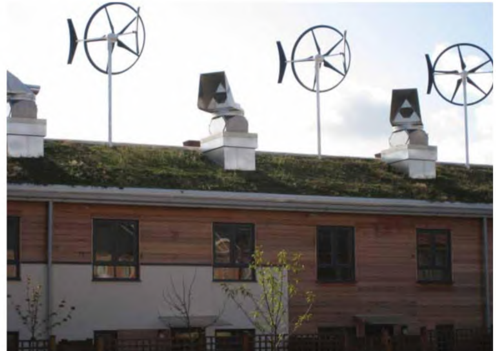
Figure 3.14 Demonstrating both energy production (wind power) and conservation (extensive type green roof)
