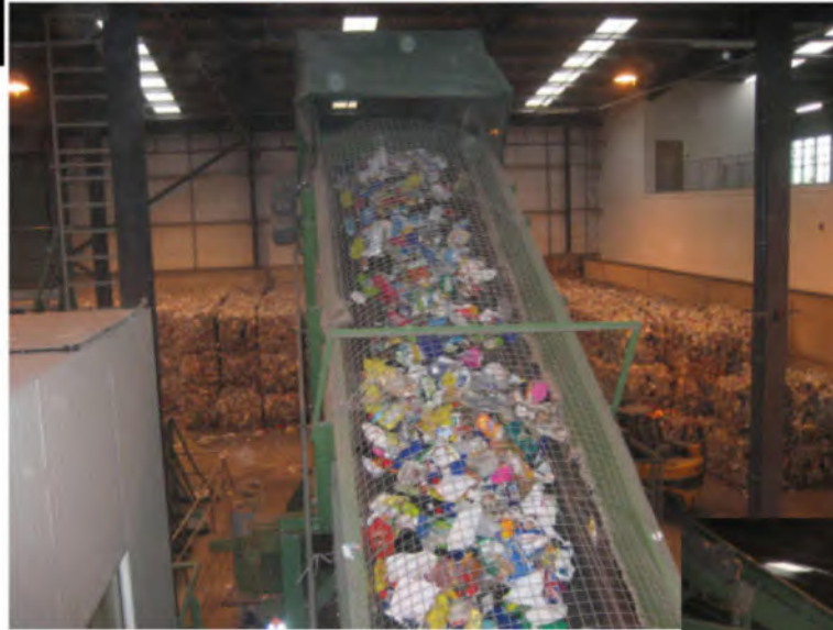
Images of the recycling process in operation at the EnviroSort facility
