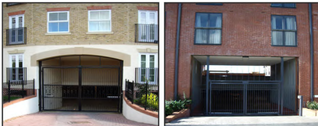
Gated entrance to underground parking with in a private residential scheme.
