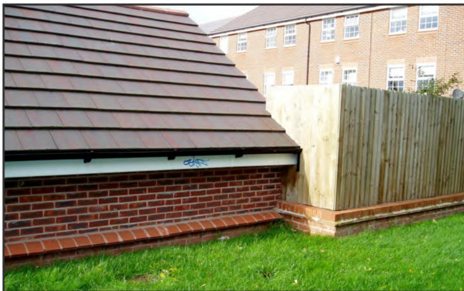
Low roofs may provide access to vulnerable areas.
