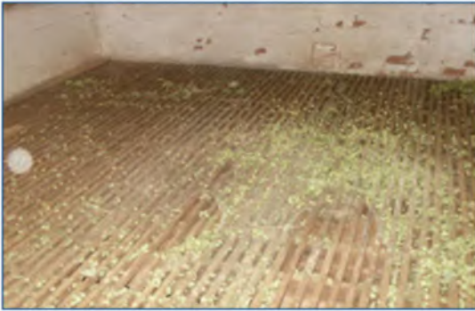
The slatted drying floor of a kiln (Herefordshire Lowlands).
