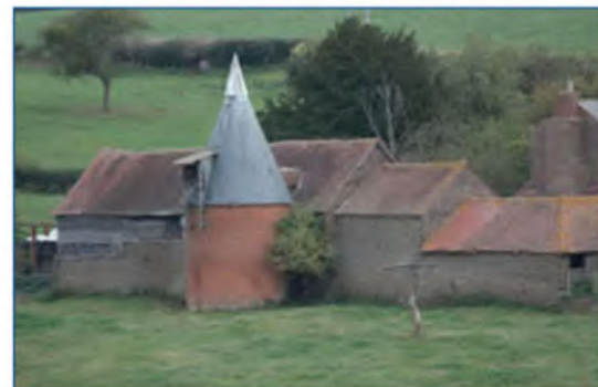
A circular hop kiln which has been added to the side of an earlier barn which was also used as the stowage (Herefordshire Plateau).
