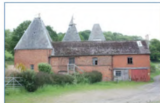
A 19th century purpose-built hop kiln and stowage. This example has three square kilns (Malvern Hills).
