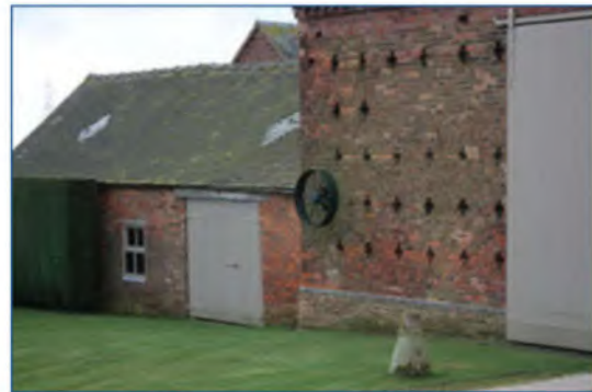
A flywheel attached to the exterior of a barn which would have been powered by a portable steam engine (Cannock Chase).
