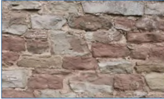
Sandstone rubble is a common material used in the west of the region.
