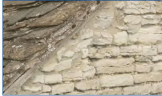
The limestone of the Cotswolds is a distinctive building material used for walling and stone slate (Cotswolds).
