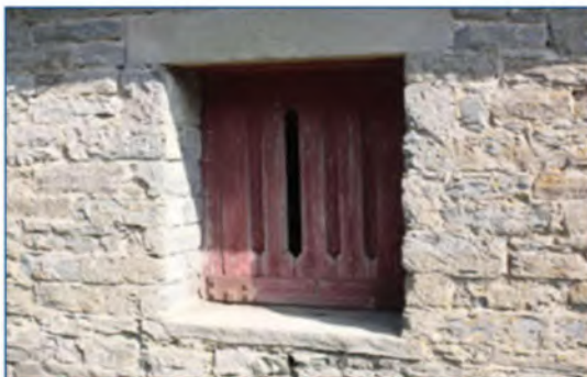
Hit and miss ventilation shutter – a characteristic feature of 19th century farm buildings (Shropshire, Cheshire and Staffordshire Plain).
