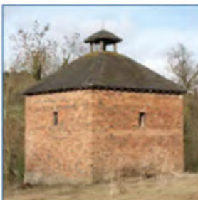
Brick-built hexagonal dovecote (Shropshire Hills).
