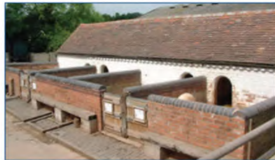
Single storey pigsties with brick-walled pens (Arden) © Peter Gaskell
