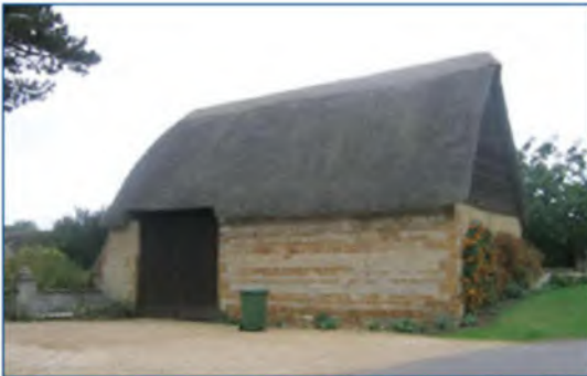
Straw thatch was a common roofing material used in arable areas but it was often replaced with plain tile or pantile. Surviving examples of thatched farm buildings are concentrated in southern Warwickshire (Dunsmore and Feldon).
