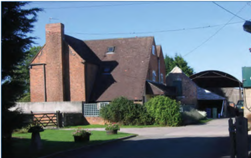
Some dairies were built as substantial additional wings, especially in dairying areas as here to the right of the farmhouse, and may have first-floor cheeserooms with loading bays (Severn and Avon Vales)
