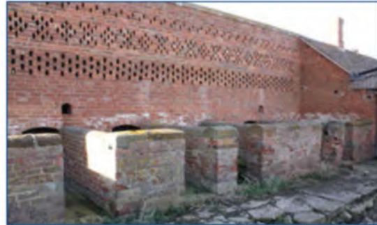
A 'poultiggery' – a series of pigsties with a hen house over forming part of a large regular courtyard farmstead on a dairy farm. The pigsties are located near to the farmhouse and dairy (Shropshire, Cheshire and Staffordshire Plain).
