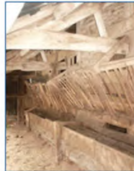
Hay racks within a shelter shed (Clun and North West Herefordshire Hills).
