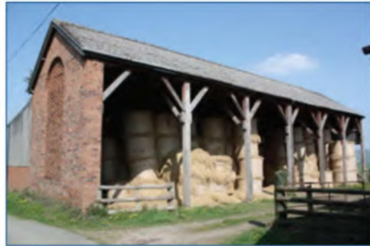
Hay barn with brick gable walls with a large panel of ventilation holes (Clun and North West Herefordshire Hills).
