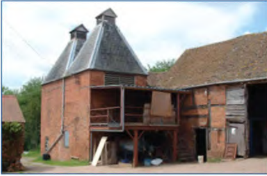
A pair of square kilns with modern staging to give access, indicating the recent continued use of the kiln for drying hops (Herefordshire Lowlands).
