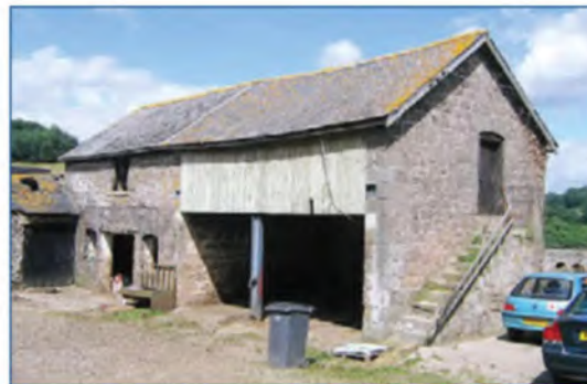
Cartshed with granary over allowing carts to be loaded directly from the granary. This cartshed adjoins a stable and faces onto a road running alongside the farmstead (Oswestry Hills).
