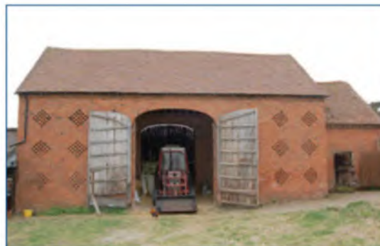
Brick barns of the 18th and 19th centuries are common across much of the region. This barn has a central threshing bay and a characteristic ventilation pattern created in the brickwork. Such barns are rarely listed (Severn and Avon Vales)
