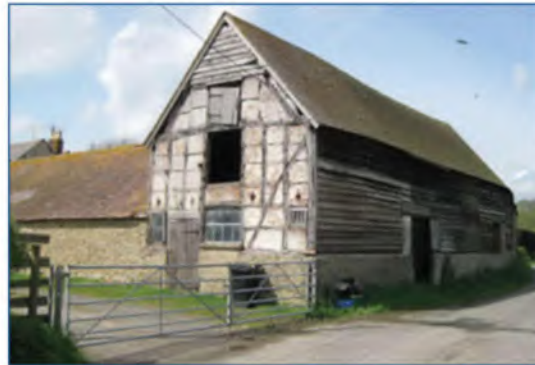
Timber-framed barns in the West Midlands typically have gabled roofs. The square panel framing of the walls is usually clad in weatherboarding or infilled with brick. Doors or openings high in the side wall may be evidence for haylofts above animal housing within the barn (Left: Herefordshire Lowlands Right: Shropshire Hills).
