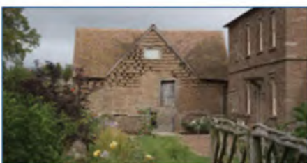
Nest boxes for pigeons were often incorporated into the gable ends of barns or, as here, stables (Herefordshire Plateau).
