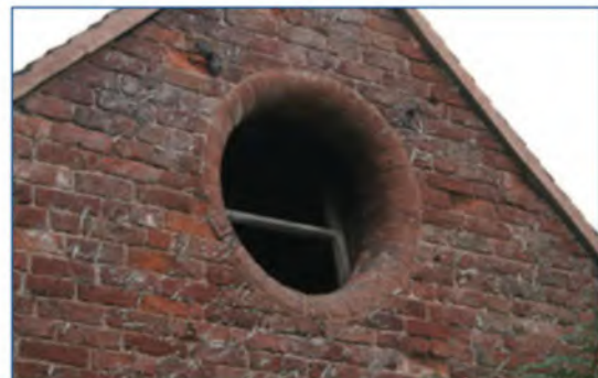
Circular pitching holes are a common feature of brick-built farm buildings, especially across lowland Staffordshire and north Shropshire (Shropshire, Cheshire and Staffordshire Plain).
