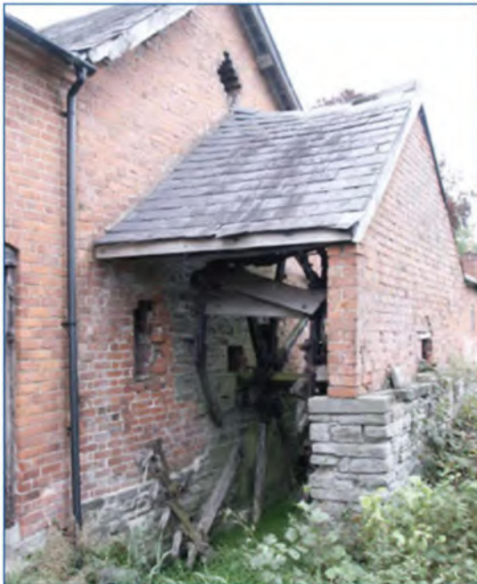
A water wheel attached to the gable end of a combination range to power threshing and mixing machinery (Herefordshire Lowlands).
