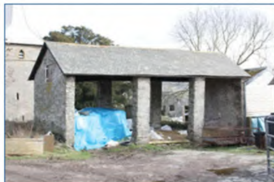
Stone-built hay barn (Shropshire Hills).
