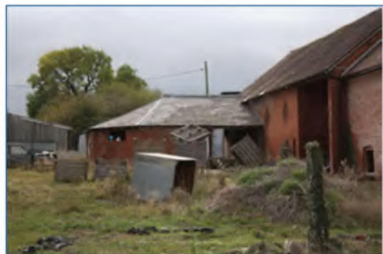
Horse engines attached to barns were more common in the arable lowland areas of the region. Such polygonal or circular buildings housed a horse engine to power threshing machinery inside the barn. Surviving engine houses are now rare and any containing machinery are extremely rare (Left: Herefordshire Plateau, Right: Arden)
