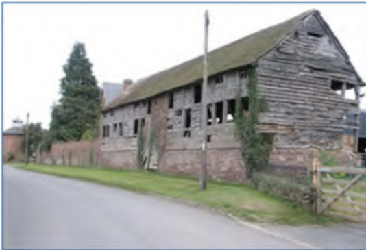
Timber-framed barns in the West Midlands typically have gabled roofs. The square panel framing of the walls is usually clad in weatherboarding or infilled with brick. Doors or openings high in the side wall may be evidence for haylofts above animal housing within the barn (Left: Herefordshire Lowlands Right: Shropshire Hills).
