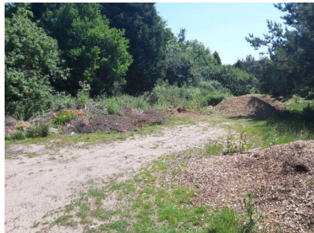
Plate 4: Access Track with Aggregate Piles
