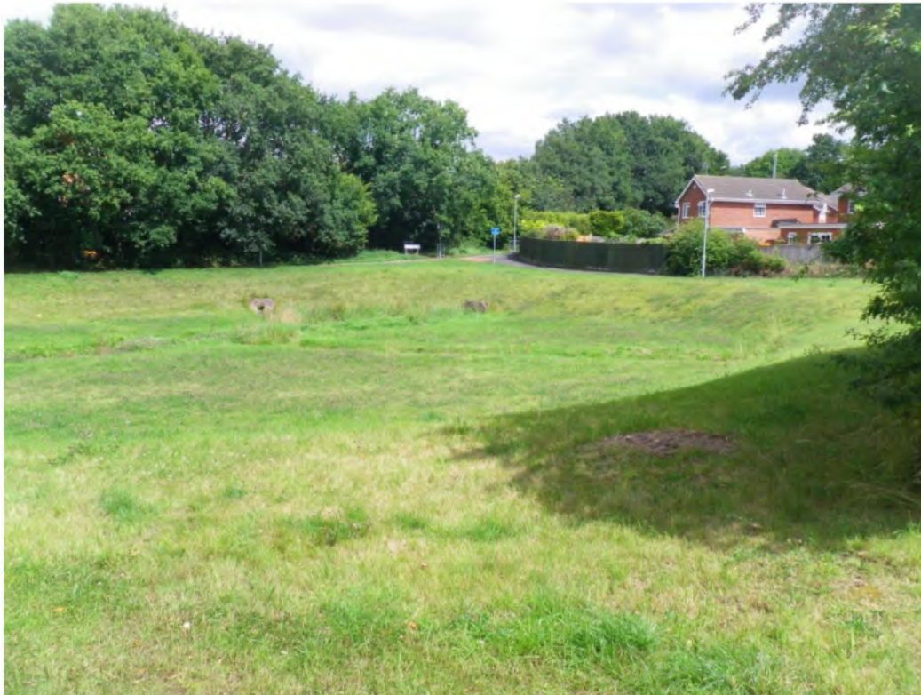
Photograph 15 - Attenuation area at upstream end of 2010/12 catchment, Church Road, Webheath
