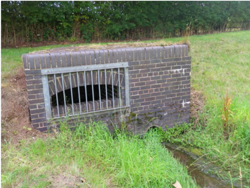
Photograph 18 - Attenuation area control structure, Church Road, Webheath
