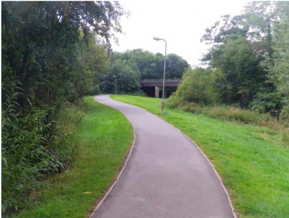
Photograph 9 - Flood defence at Paper Mill, Brooklands Lane, looking downstream, house to left
