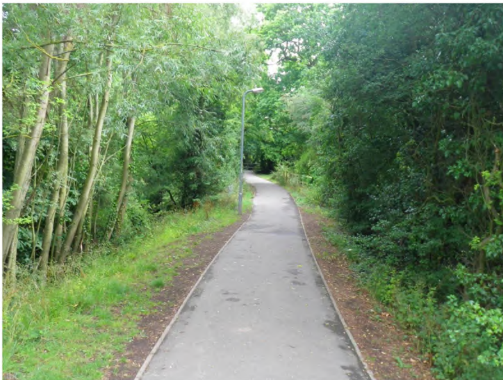
Photograph 10 - Flood defence at Paper Mill, Brooklands Lane, looking upstream
