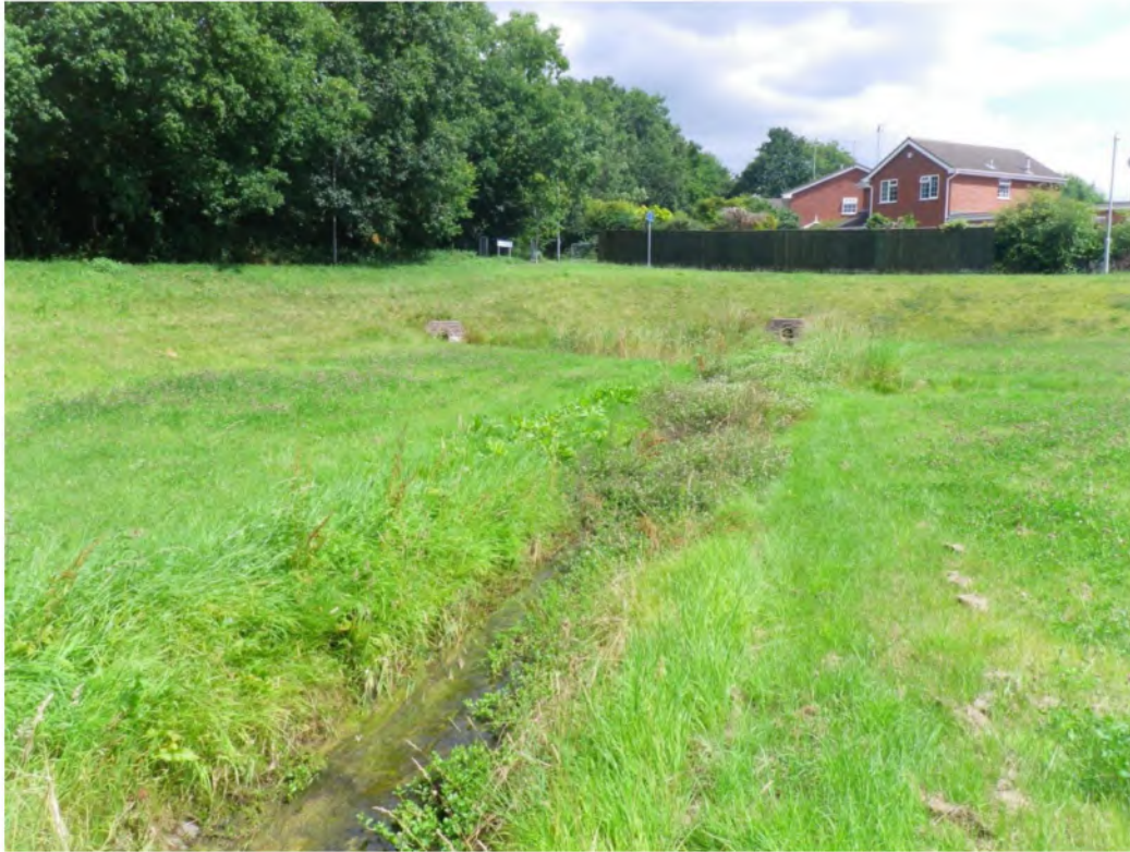
Photograph 19 - Attenuation area control structure, Church Road, Webheath
