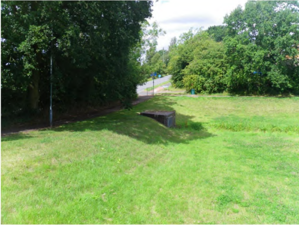
Photograph 17 - Attenuation area at upstream end of 2010/12 catchment, Church Road, Webheath
