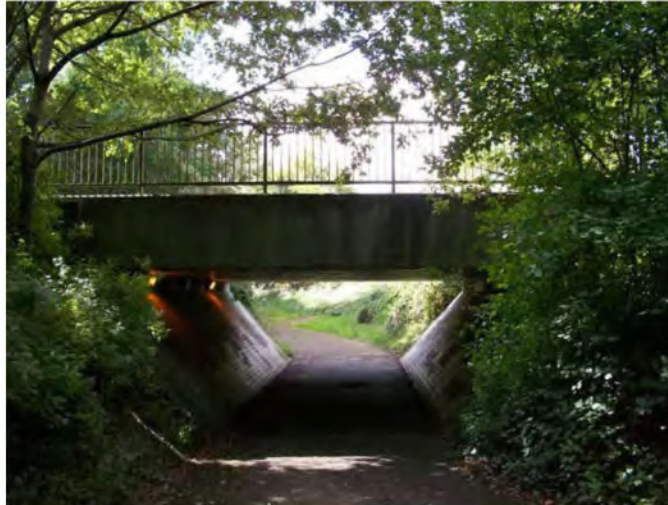
Plate 9 – Typical underpass under Far Moor Lane
