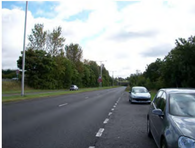
Plate 4 – A4023 Coventry Highway adjacent to Development Site
