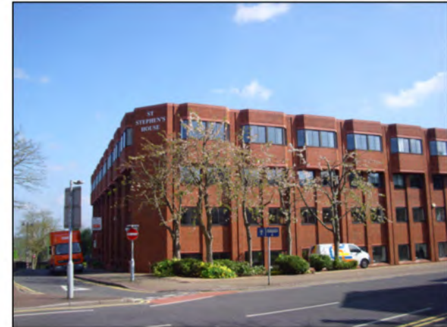
Photograph 3.2: St Stephen House – Office Development
