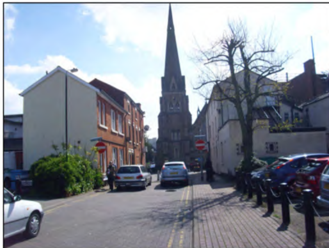
Photograph 4.8: View of St Stephens Church
