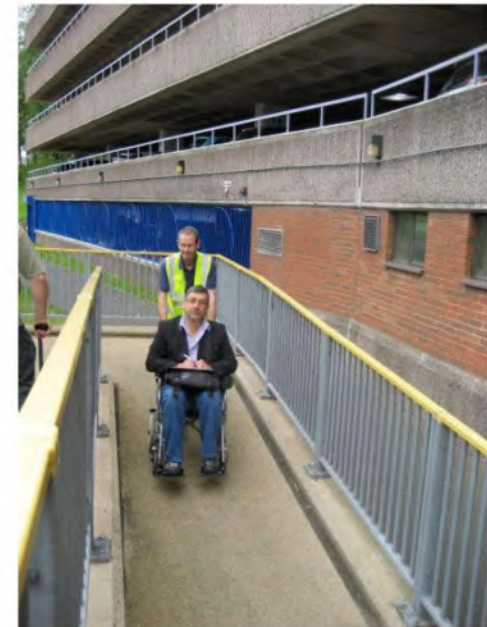
Figure 2: Dial a Ride customers access Shopmobility using a ramp located immediately beside the vehicle stopping point. The ramp uses an “anti-slip” surface which is designed to minimise the risk of customer falls.
