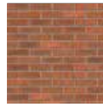
Main Facade / Plinth Ibstock - Weston Red Multi
