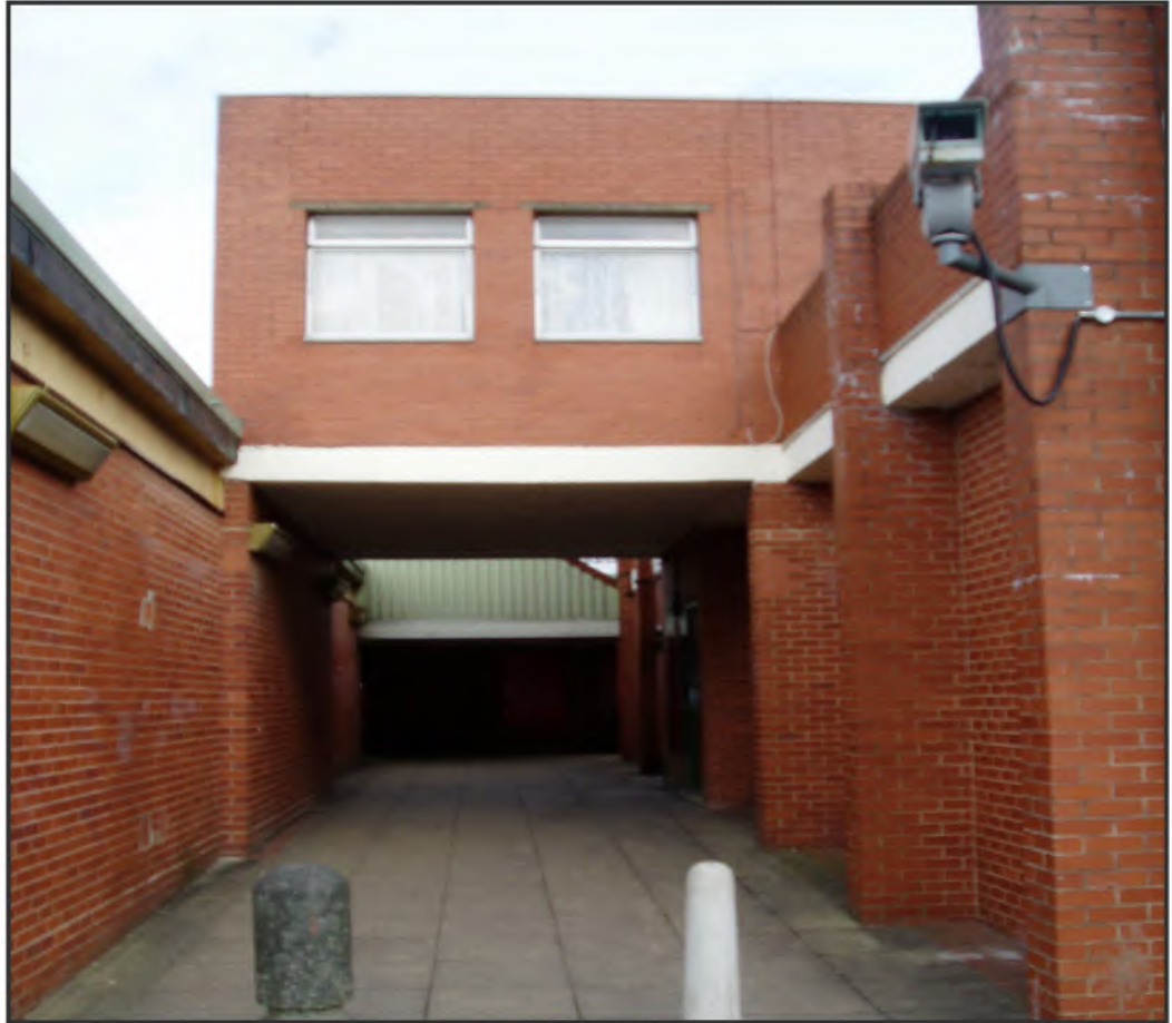
Secluded and covered entrances lack natural surveillance.
