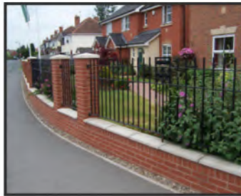
A visually permeable physical boundary.
