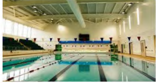
Abbey Stadium Sports Centre Pool
