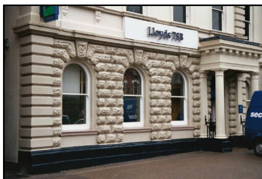
Fig 26: Rock faced rustication No 19 Church Green East
