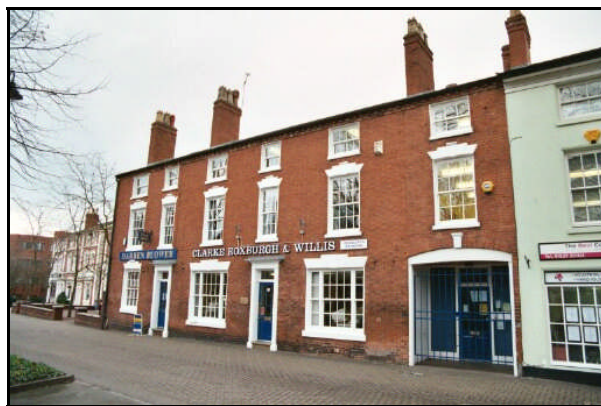
Fig 19: Church Green East looking North
