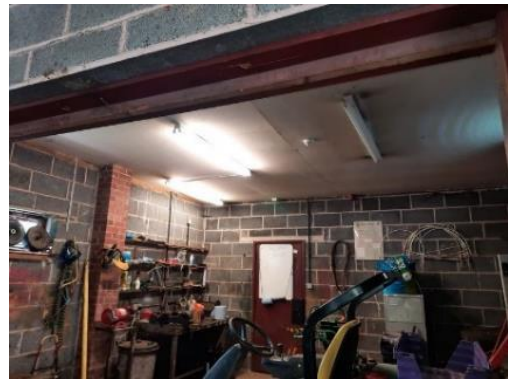
Plate 4.15: Section of building with inaccessible roof void
