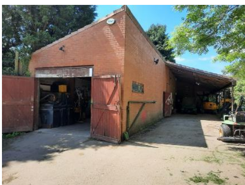
Plate 4.1: Eastern and northern elevations
