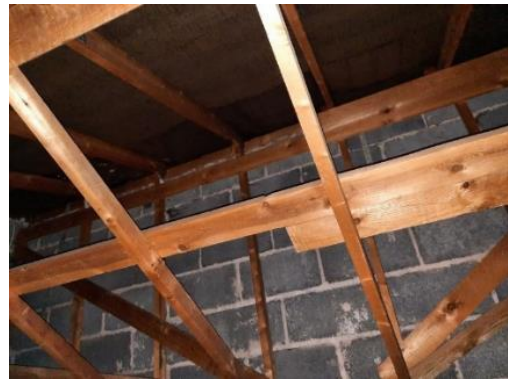
Plate 4.13: Roof structure above offices
