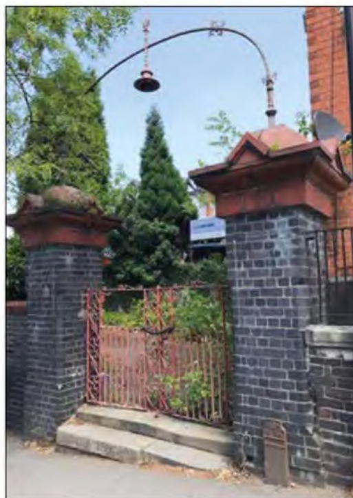
Cast iron light fitting above the entrance to the Methodist Chapel and Manse
