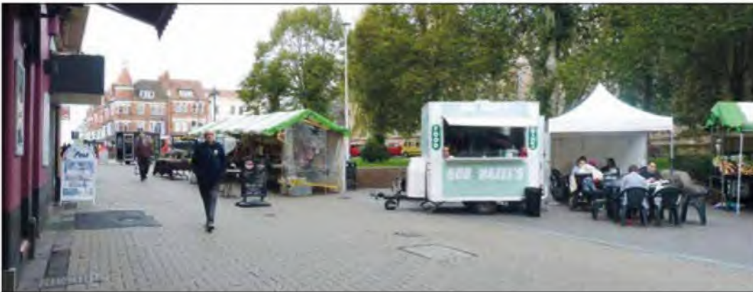
Expanse of block paving on Market Place
