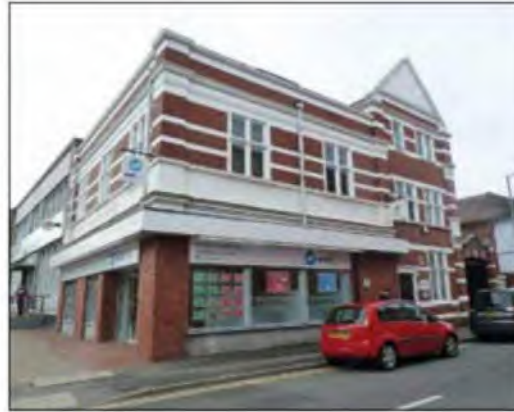
County House, corner of Church Green West and Church Road
