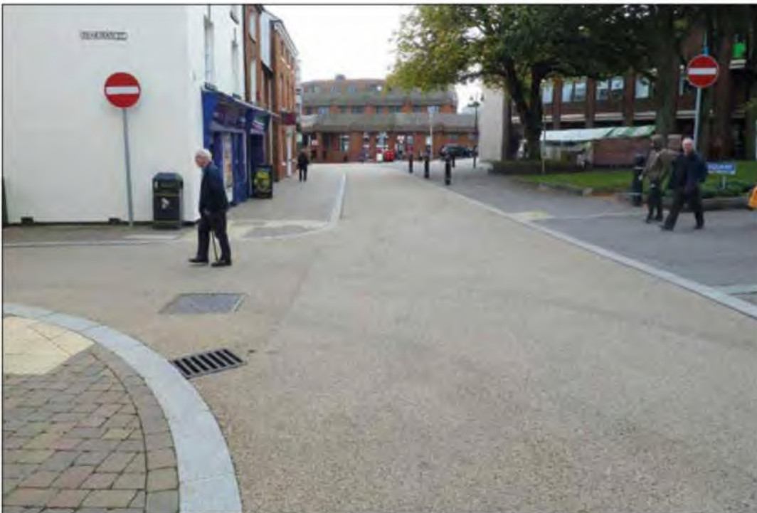
Part of the new public realm scheme at the junction of Church Green West and Peakman Street
