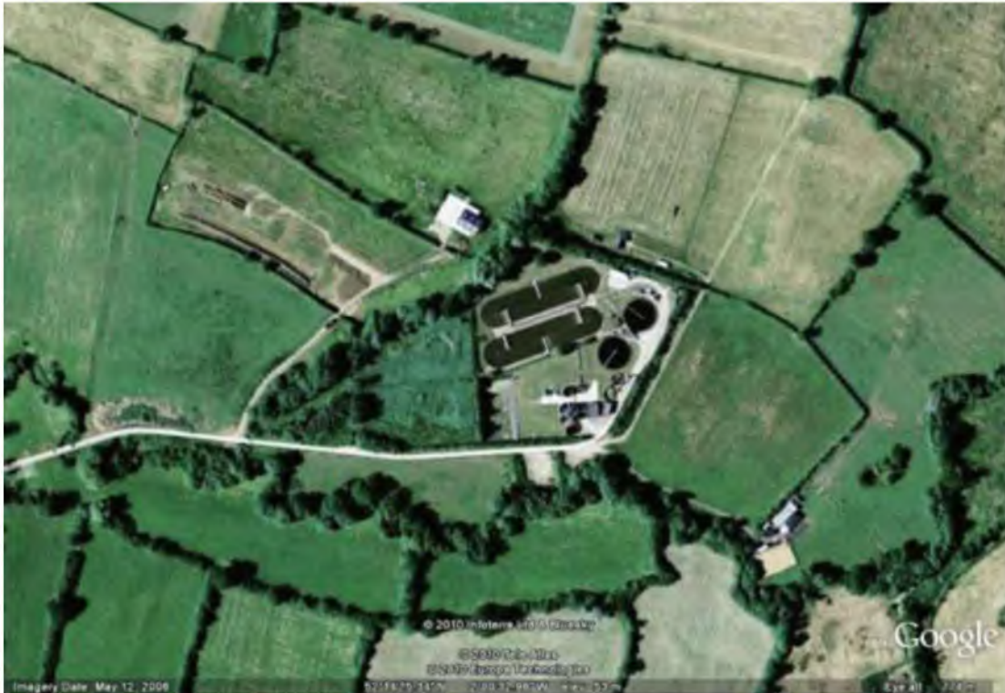
Figure 7-2 Aerial Image of Priest Bridge STW
