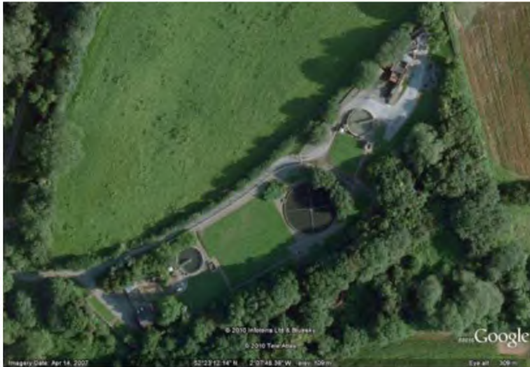
Figure 7-5 Aerial Image of Belbroughton STW
